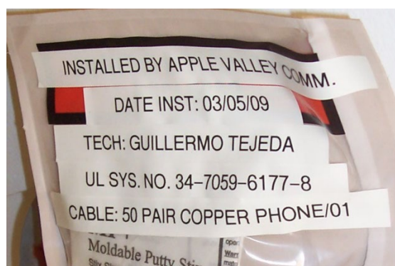
Figure 2-9. Firestopping Label – Example
